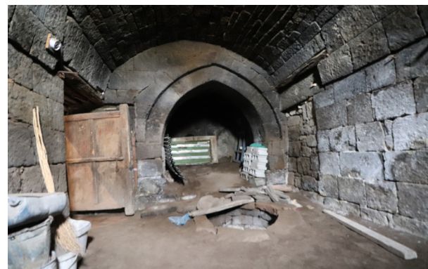
Fig. 3 - The kitchen and cooking pit, ground floor
