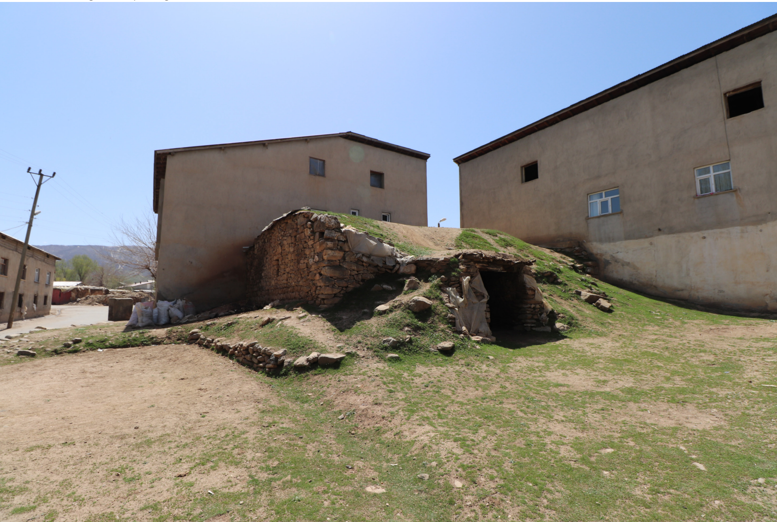
Fig. 1 - Surp Giragos Church, northeastern view
