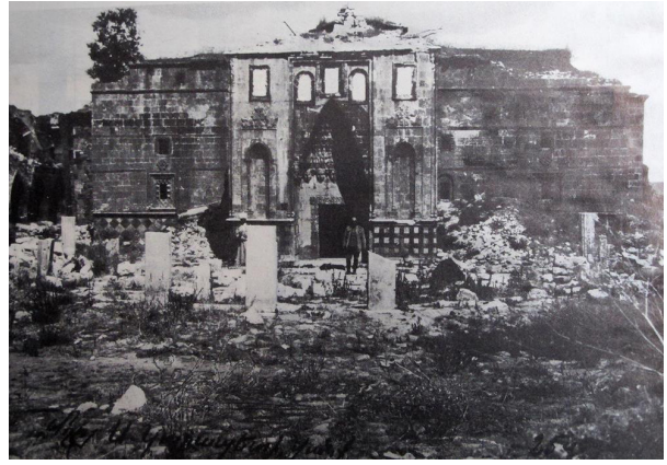
Fig. 5 - Collapsed Bell Tower and western façade of the mother church complex after 1915 (Thierry 1983, 401)
