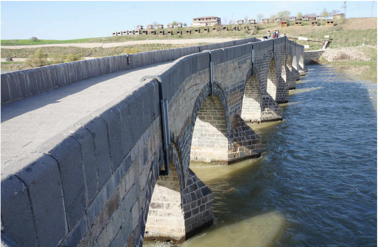
Fig. 3 - Cutwaters of the bridge facing the upstream direction
