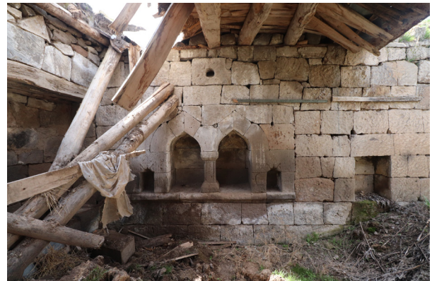
Fig. 4 - The masonry structure in Mollakent cemetery, the organization of niches among the ashlar coursing
