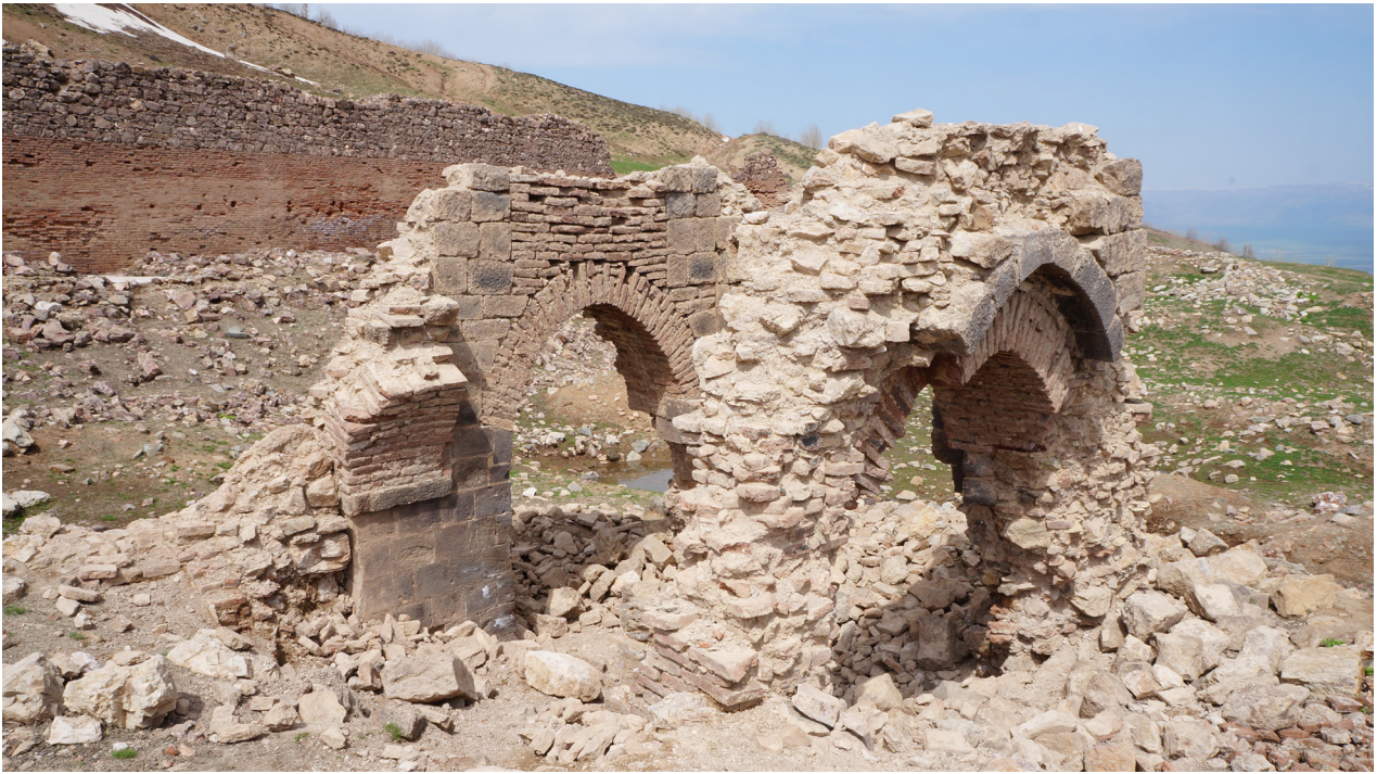
Fig. 3 - Transition space with arches
