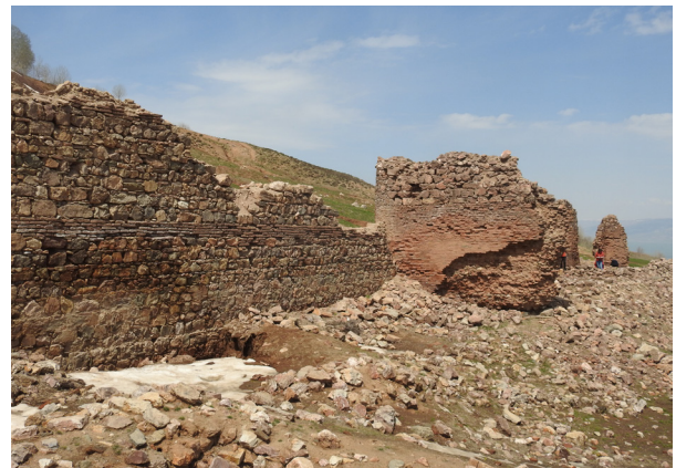
Fig. 4 - Western fall extending north-south, various coursing methods
