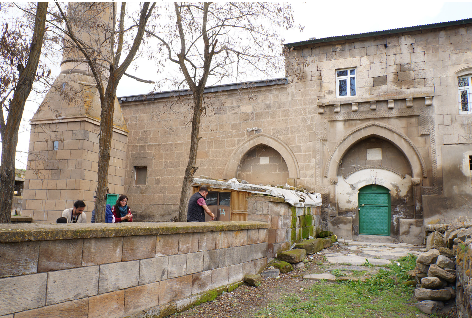
Fig. 1 - Eastern view of Mollakent Mosque and Divan Mansion
