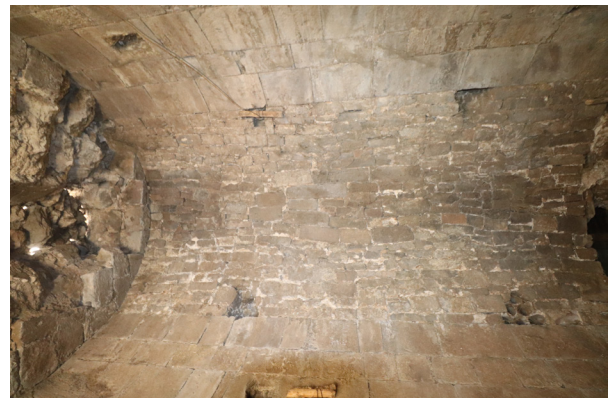
Fig. 6 - Vault and acoustic amphorae
