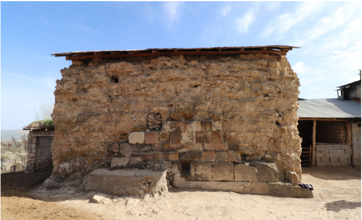
Fig. 3 - Surp Sahak Church, northern façade
