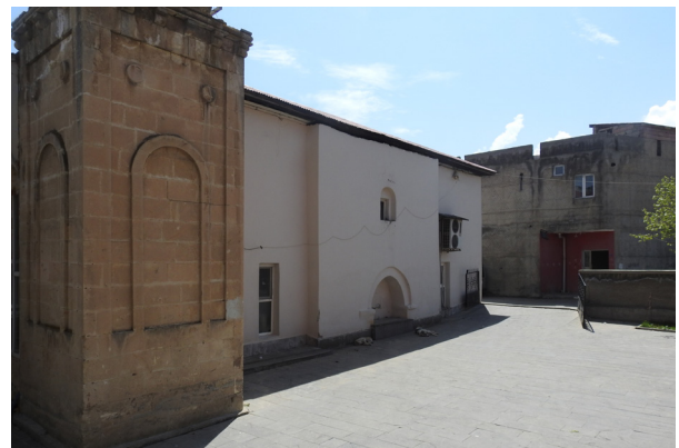
Fig. 4 - Pedestal of the minaret and the western wall
