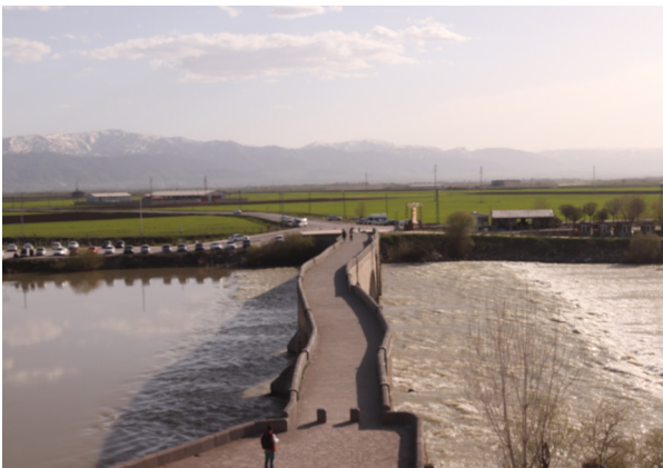
Fig. 4 - Murat Bridge, southwestern view
