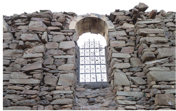
Fig. 6 - Detail of iron window bars
