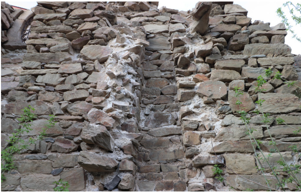
Fig. 5 - Detail of chimney
