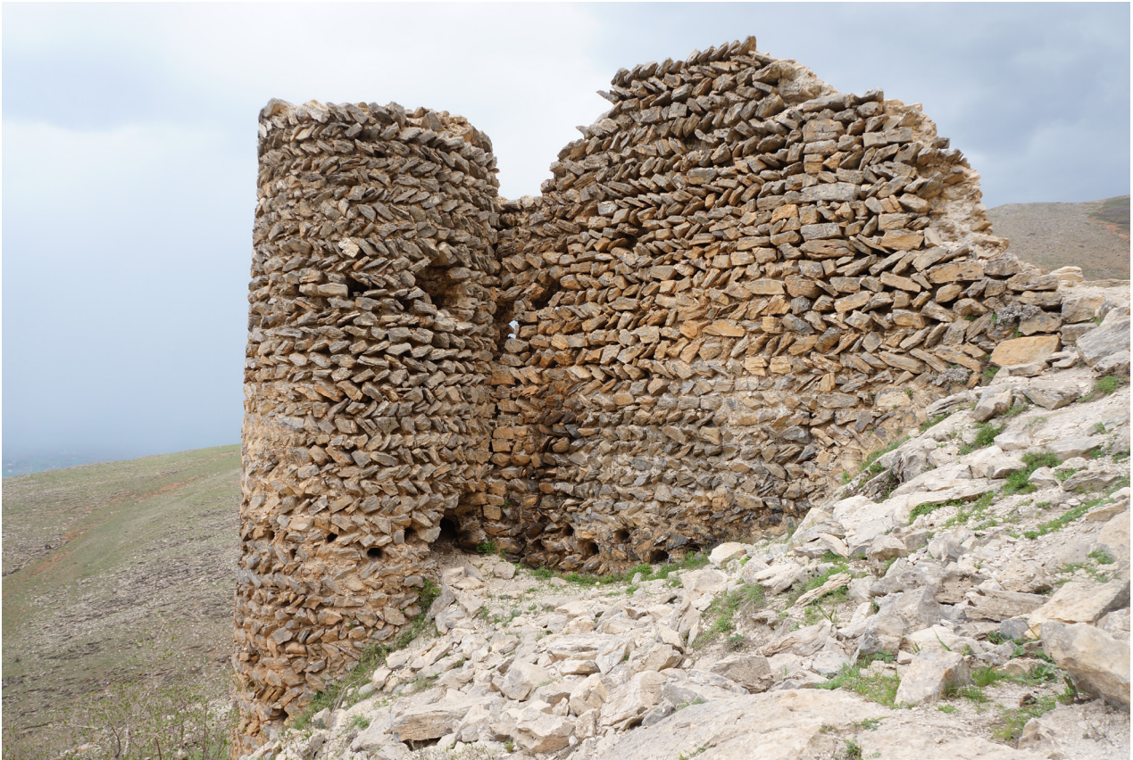
Fig. 2 - Herringbone masonry in the Fortress of Haspet
