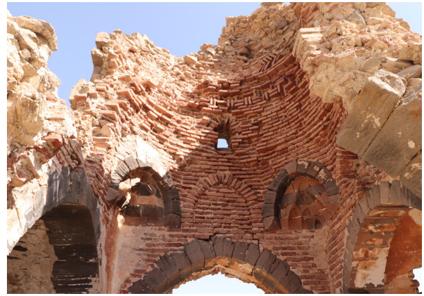
Fig. 11 - Corner squinch embellished with muqarnas
