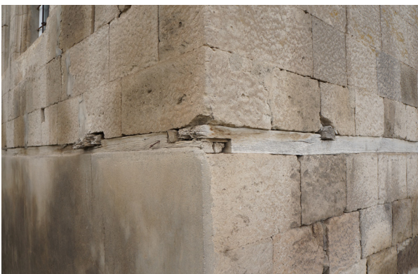
Fig. 8 - Joint between wooden lacing
