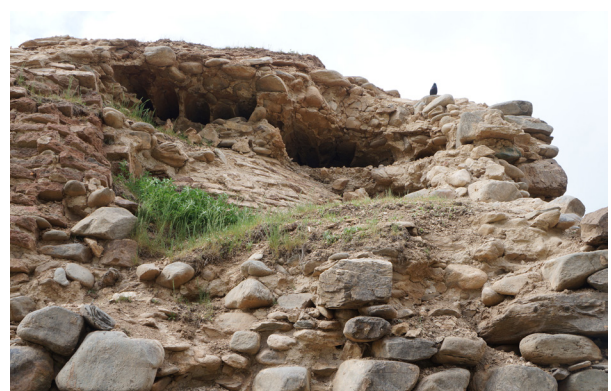
Fig. 5 - Detail, infill of the hemispherical dome above the apse
