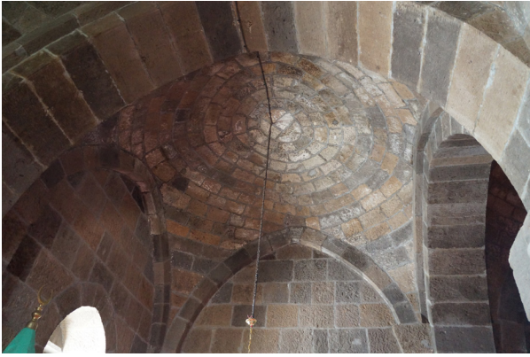
Fig. 3 - Detail of a dome and its pendentives
