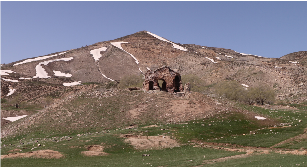
Fig. 5 - Surp Arakelots Monastery, view from the east
