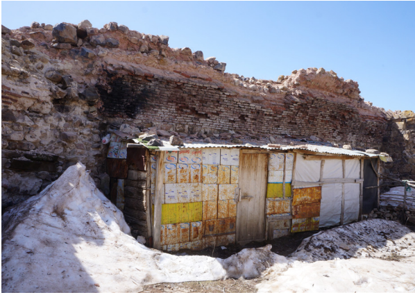
Fig. 13 - Surp Kevork Church, southern wall, view from the northeast
