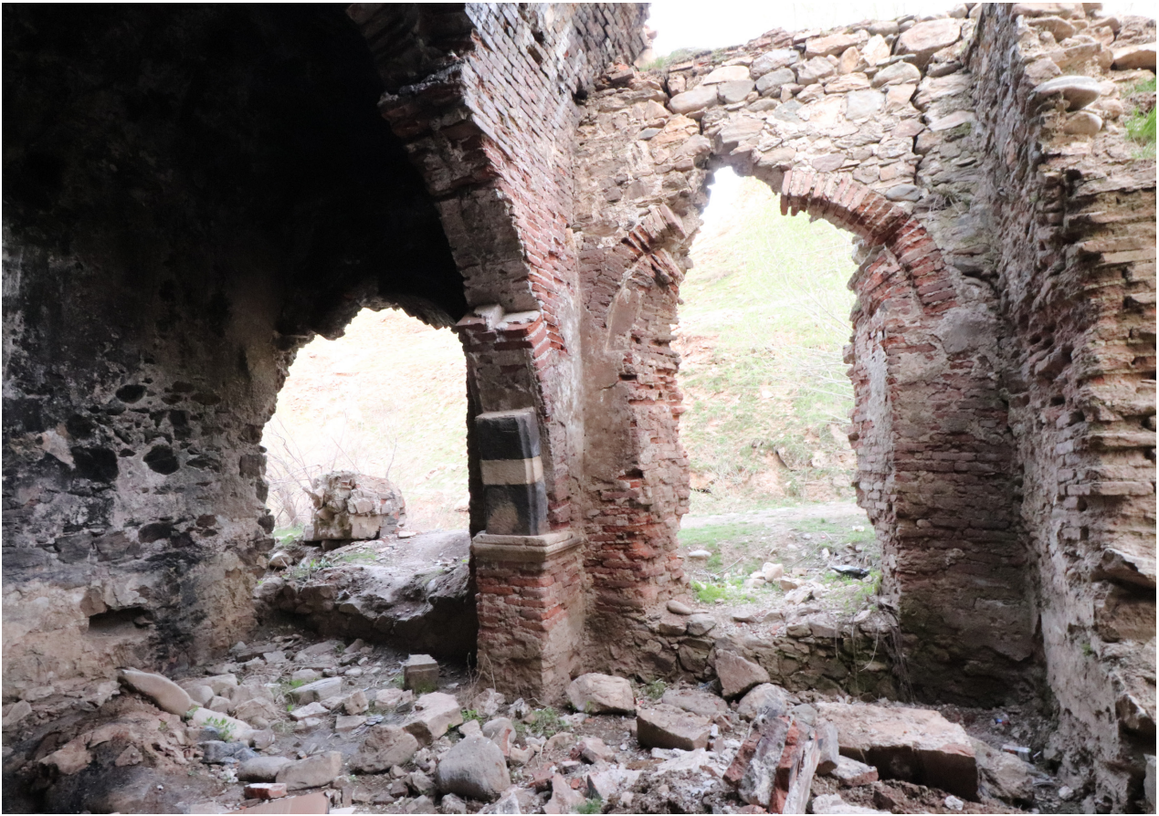
Fig. 3 - Coloured-stone and brick masonry
