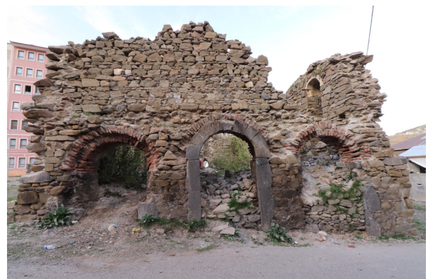
Fig. 4 - Southwestern entrance and traces of lacing
