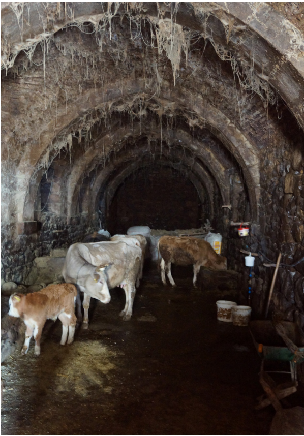
Fig. 14 - The old guesthouse building, currently used as a barn
