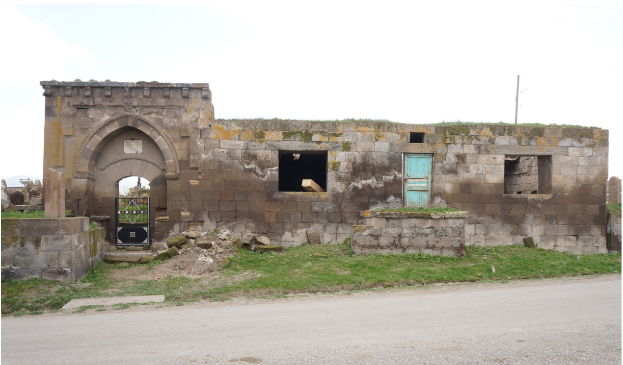
Fig. 3 - Mollakent cemetery, entrance portal and adjoining masonry structure, northern façade
