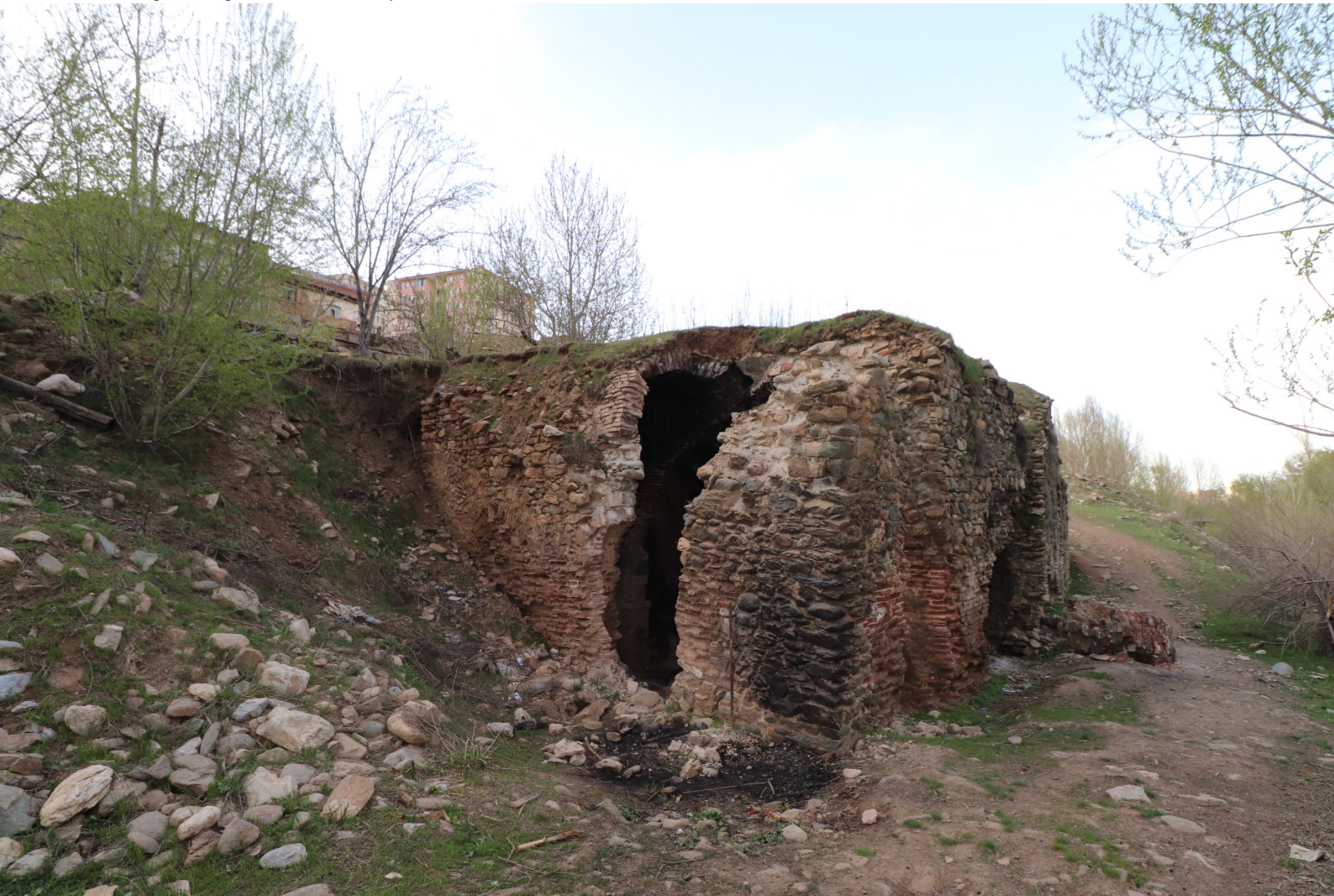
Fig. 1 - Migre Bathhouse, view from the southeast
