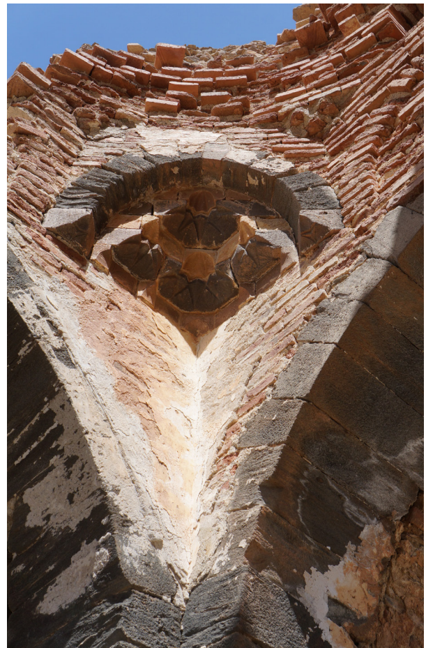
Fig. 12 - Window and interlocked brick masonry
