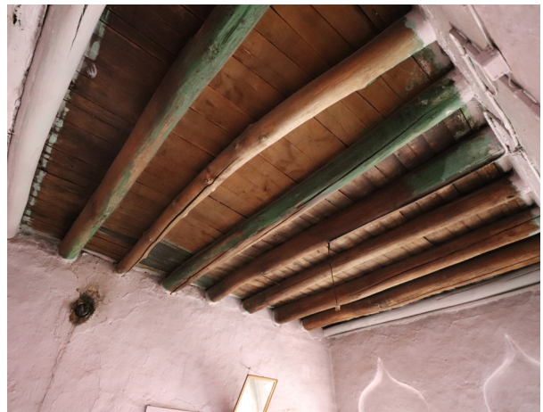
Fig. 7 - Circular, wooden beams supporting the flooring
