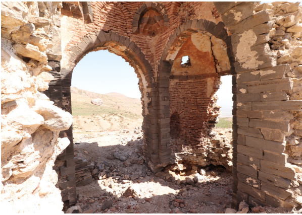
Fig. 10 - Ashlar-stone and brick masonry units
