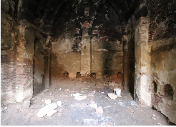
Fig. 4 - View of the steam hall
