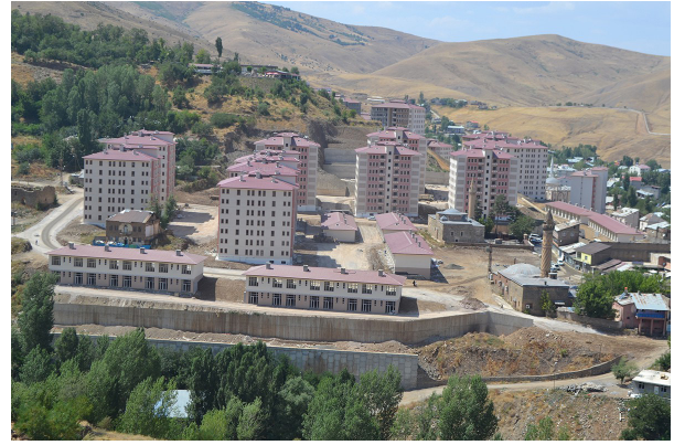
Fig. 3 - View of Kale Neighbourhood following the demolition and construction. Photograph: Bekir Avcı
