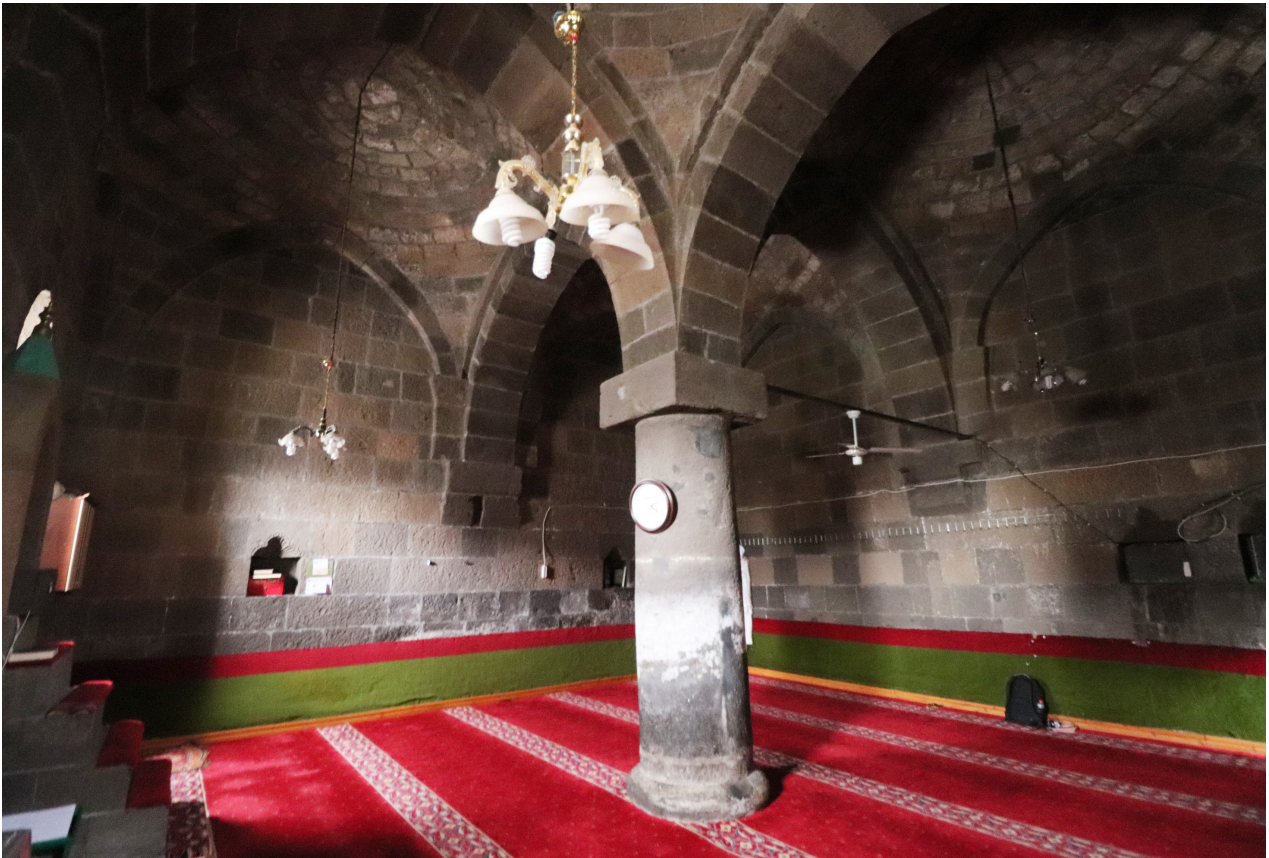
Fig. 2 - The interior, with the column supporting the four domes
