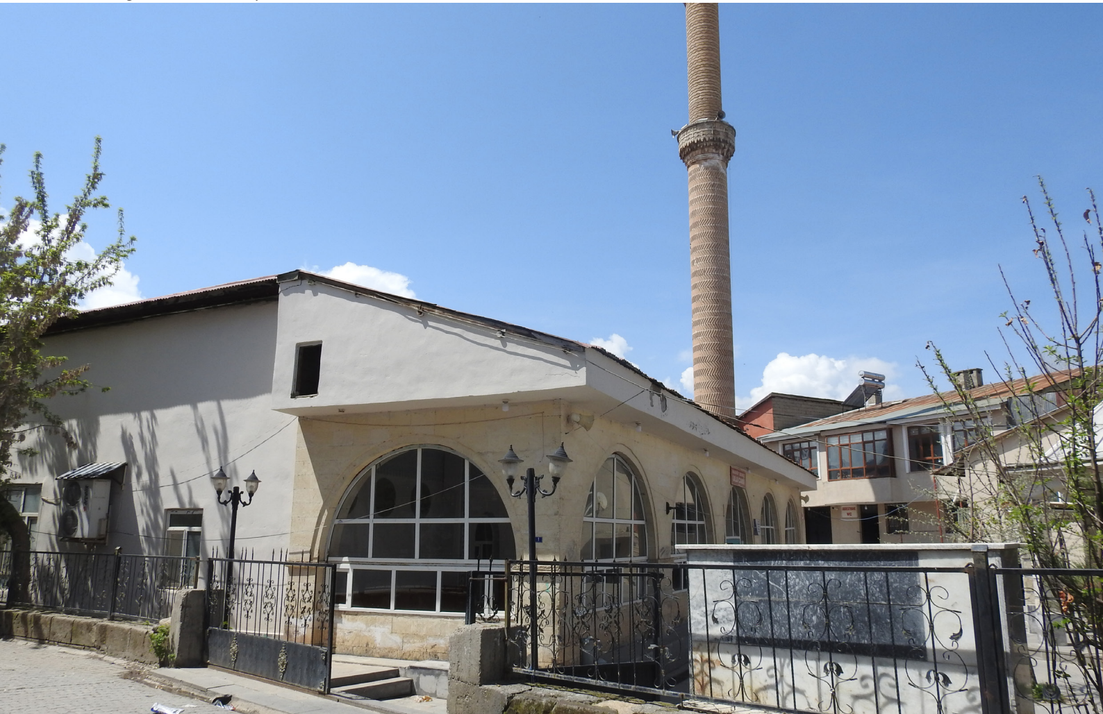
Fig. 1 - General view from the northeast
