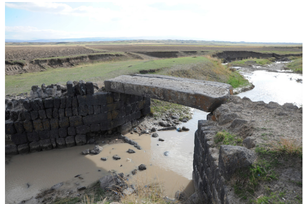
Fig. 3 - Kız Bridge, before the restoration, 2014
