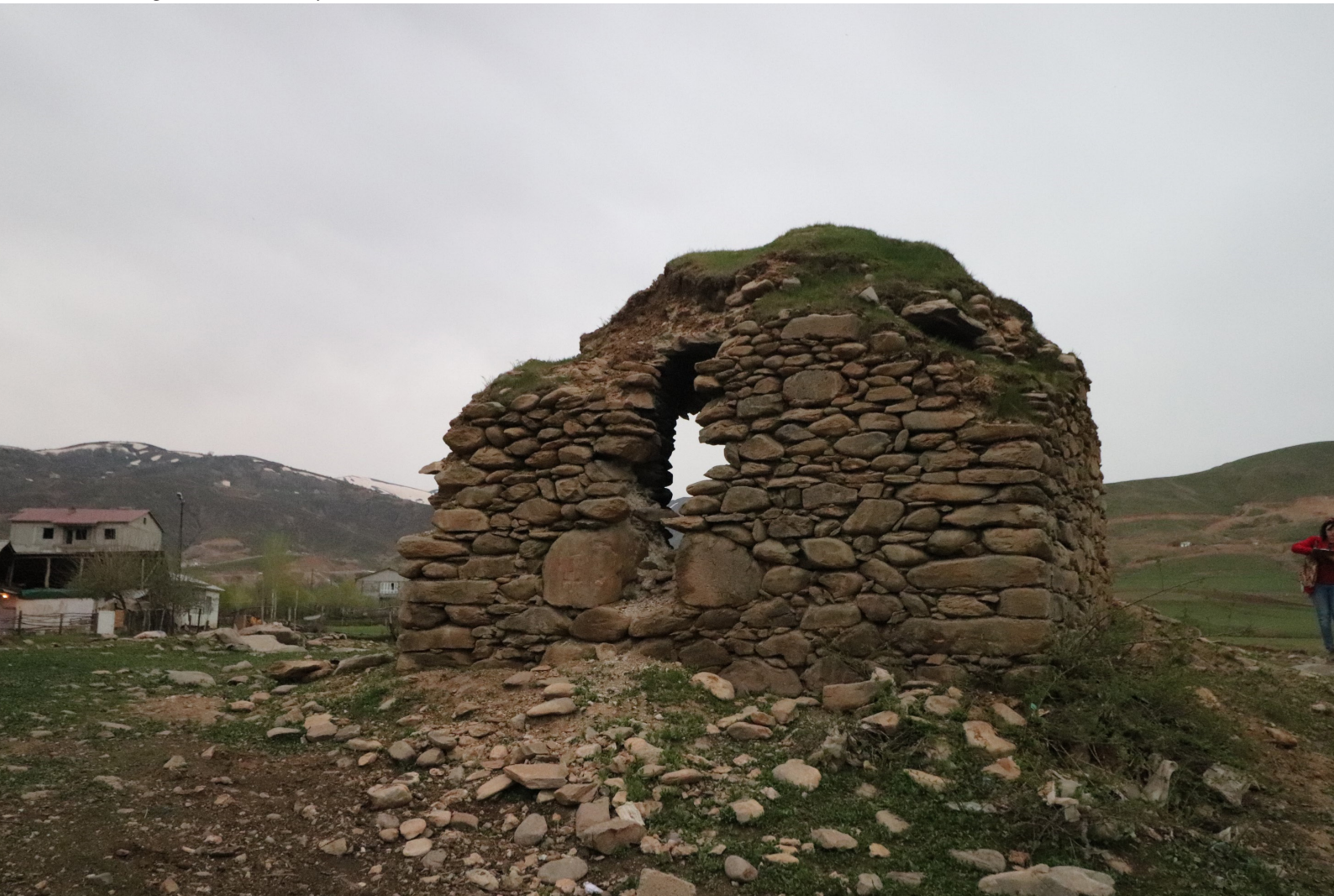
Fig. 1 - Eastern view of the structure and environs
