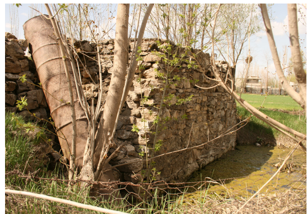
Fig. 5 - Drainage pipe, eastern view
