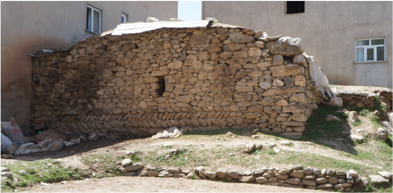
Fig. 3 - Eastern façade and rubble coursing with herringbone pattern
